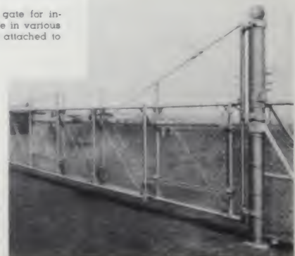
The Cyclone gate below was developed especially for large, busy airports. It is a combination of Swing and Roller gates in one installation. Doesn't the huge post at the extreme right appear solid enough to support even this mammoth gate with ease?
